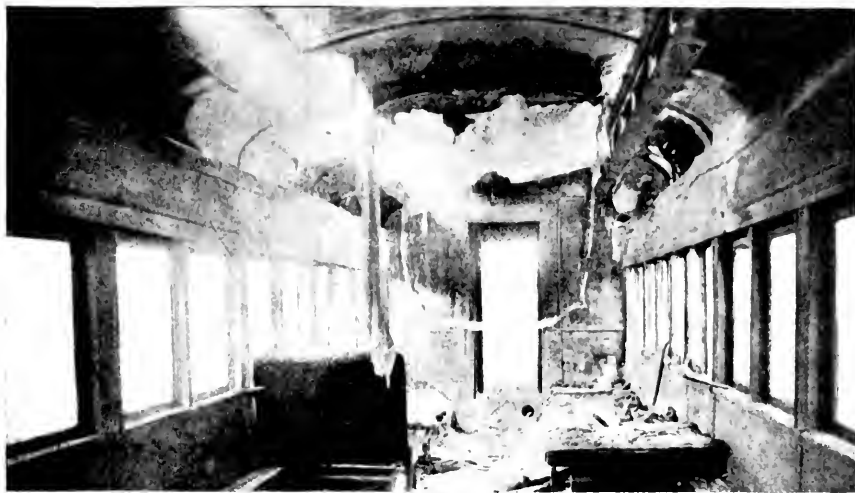
Interior of Steel Passenger Car after Fire Test
